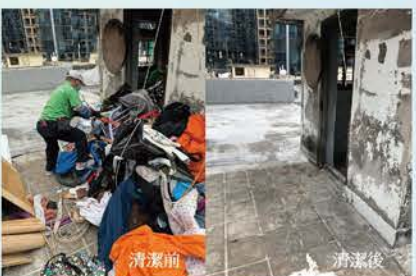
A cleansing contractor commissioned by the Yau Tsim Mong District Office cleansed the rubbish accumulated inside the common parts of "3-nil" buildings.
